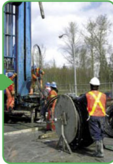
■ Lowering of geo loop.
