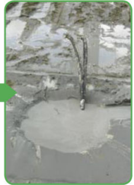
■ Completed geo loop installation.
